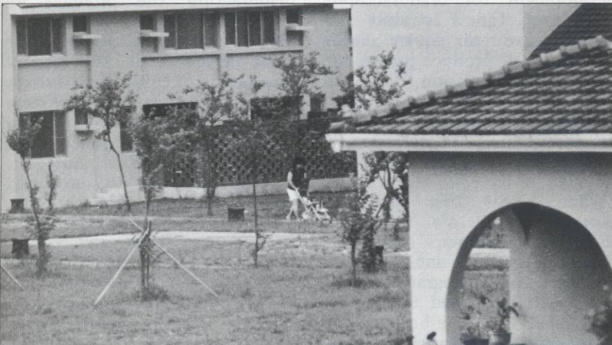
Housing for Park workers.
